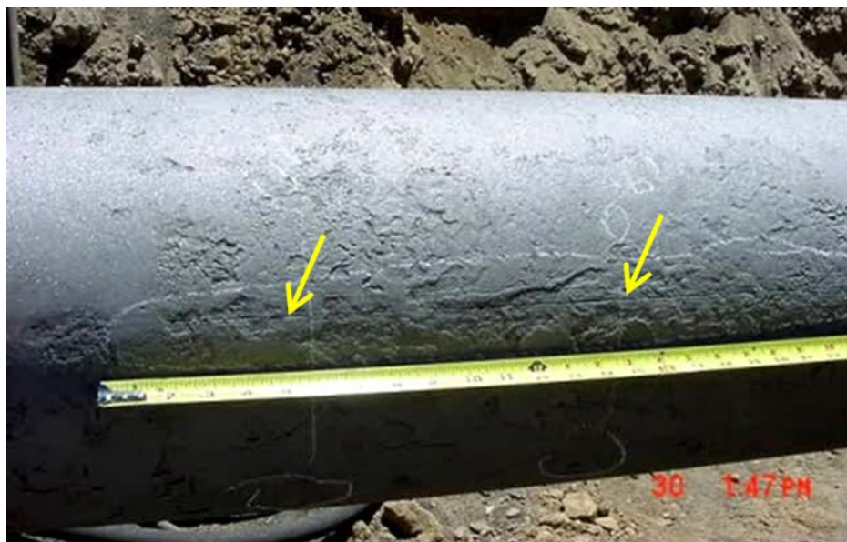
Figure 8. Typical external appearance of selective seam weld corrosion
