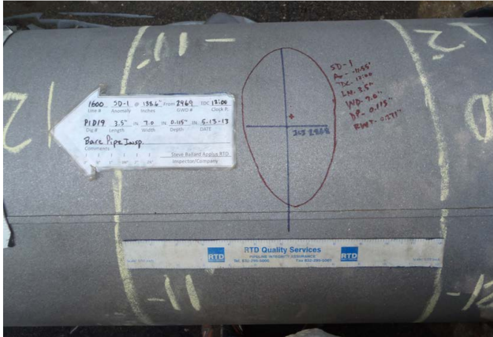
Figure 5. External Appearance of the Flash Welded Pipe Seam on Line 1600
