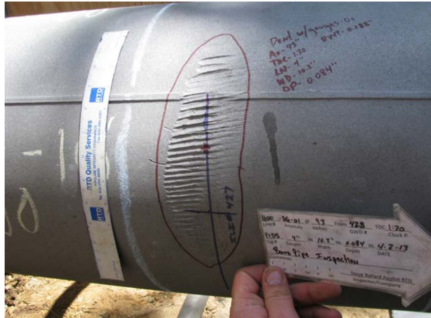
Figure 10. Prior Mechanical Damage Discovered on Line 1600
